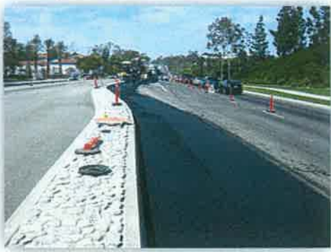
Golden Lantern Roadway Widening
