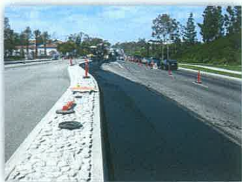
Golden Lantern Roadway Widening City of Laguna Niguel
